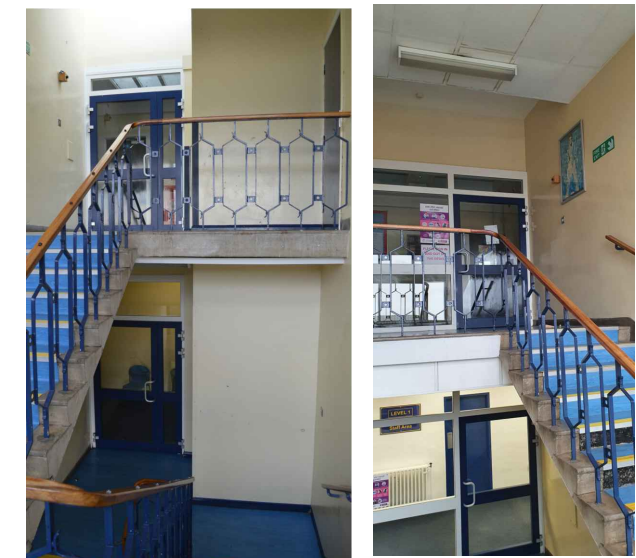
Staircase in main teaching block
